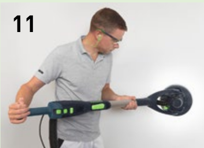
Sand down the filled wall using the Festool PLANEX LHS 2 225 long-reach sander and the Granat Net P120-P180 abrasive.
