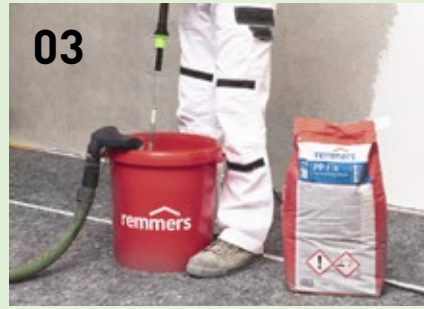
Mix PP Fix, an adhesive mortar for mould remediation, using the Festool MX 1200 stirrer and the HS3L mixing container.
