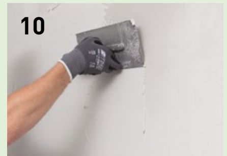
Mix iQ Fill fine plaster and fill. When hardened, the plaster is permeable and water-resistant.
