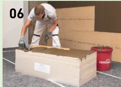
For full-surface adhesion of insulation panels, PP Fix is applied to the wall and panel using a toothed trowel.
