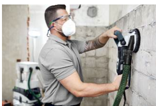
Image: Festool-RG130ECI-17.jpg The brush ring adapts to the surface being sanded and therefore ensures excellent extraction.
